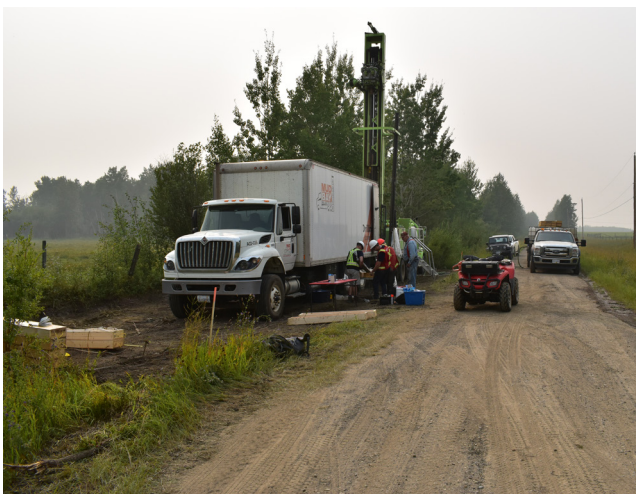
Drillers install monitoring wells at the Hudson's Hope Station
