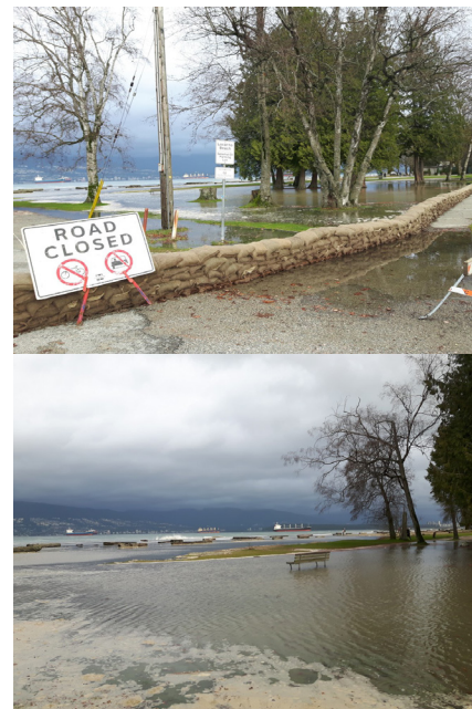
Flooding at Vancouver's Locarno Beach during the Dec. 20, 2018 storm surge
